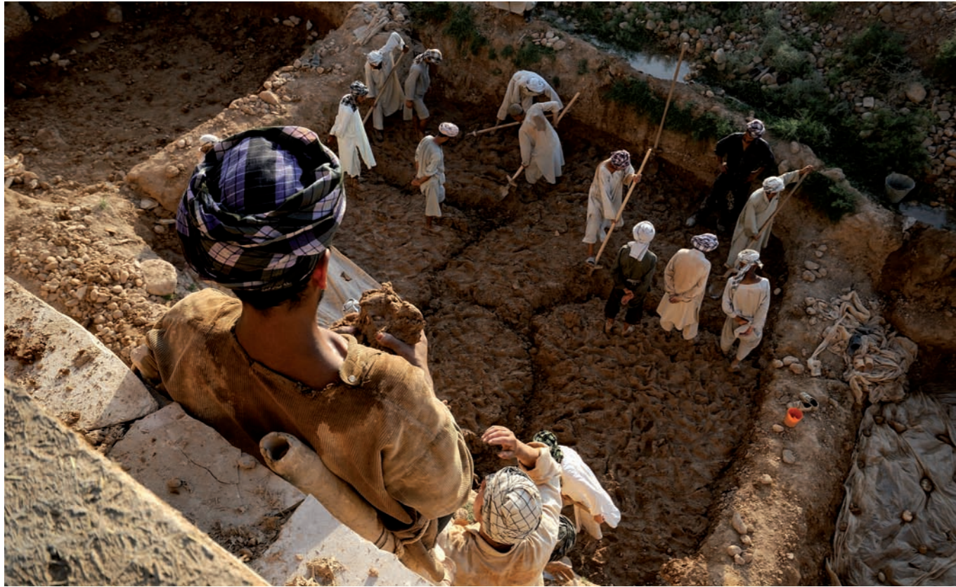
The pakhsa is made in special fields for the traditional reconstruction of the garden walls of the Bagh-e Jehan Nama Palace.
