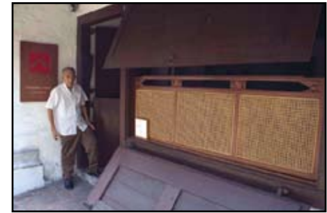
fig. 10, A local initiative to restore a Dutch House at the 8 Heeren Street Malacca, Malaysia
