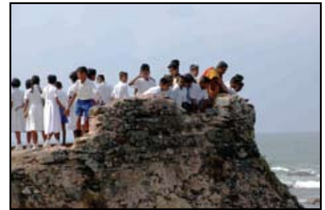
fig. 23, Flagpoint Galle, Sri Lanka before restoration.
