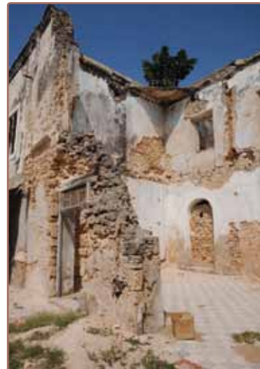
Endangered heritage Ilha de Mozambique
